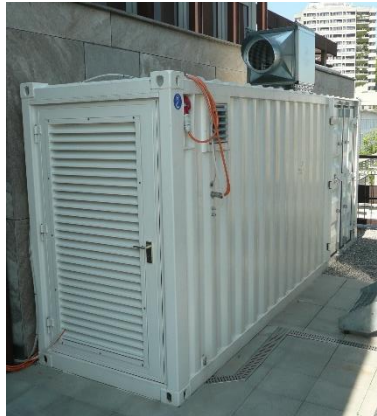
Direct Air Capture Unit
